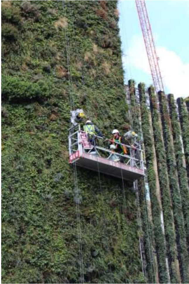
Figure 1: Maintenance of exterior vertical green walls Source: Sabina Šegula, London, 2016
