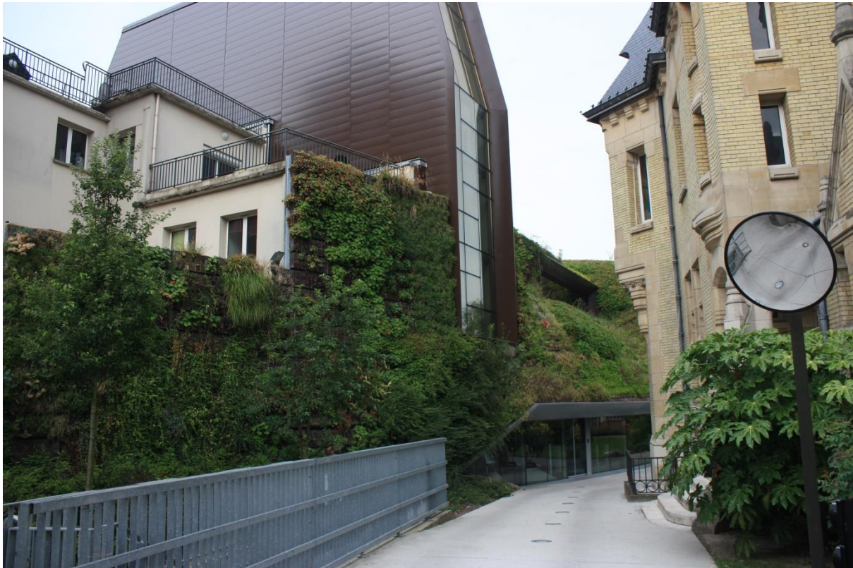
Slika 8: Zelena stena po sistemu Tracer Vertiflore, Amiens Chamber of Commerce (FR) Source: Sarah Milliken
