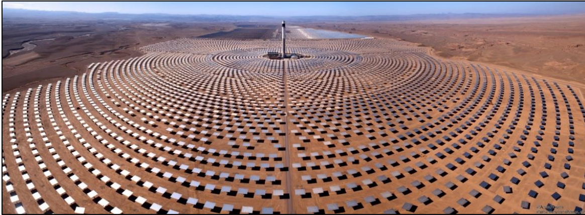
Figure 9: Noor Solar Power Station 9
