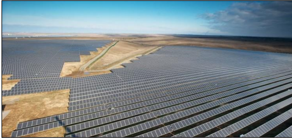
Figure 16: Benban Solar Park 17
