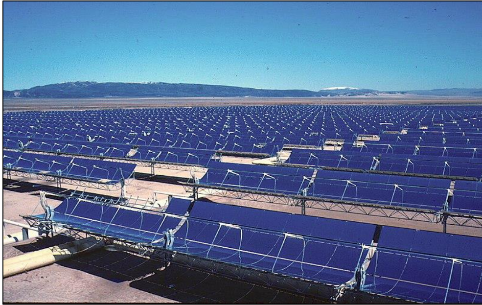
Figure 11: Solar Energy Generating Systems (SEGS) 11
