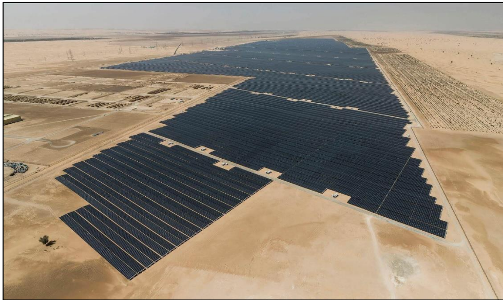
Figure 17: Benban Solar Park 19
