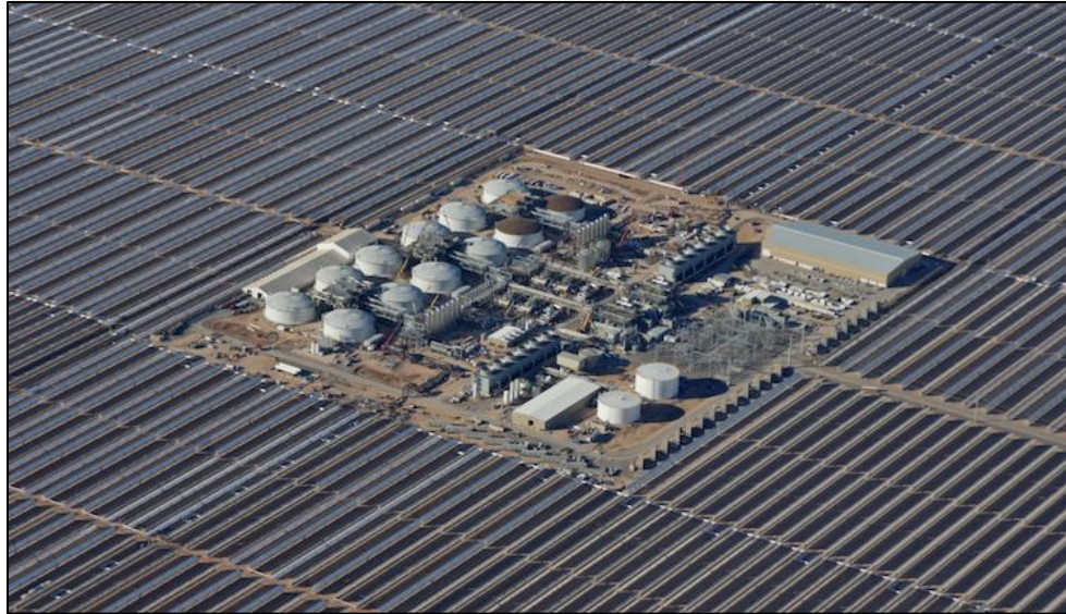
Figure 13: Solana Generating Station 13
