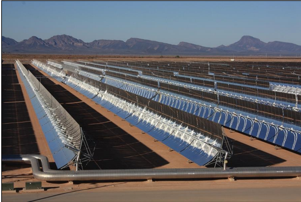
Figure 12: Mojave Solar Project 12
