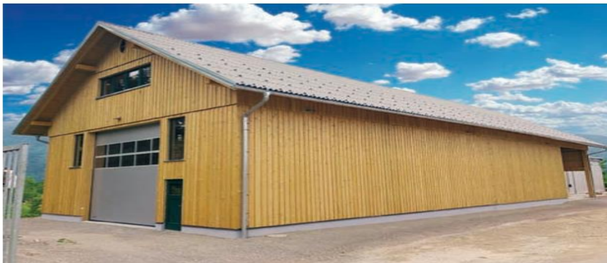
Picture 3. Air-conditioned storage space with two wood-dryers. Source: (Gjerkeš, 2020)
