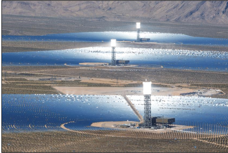
Figure 10: Ivanpah Solar Power 10
