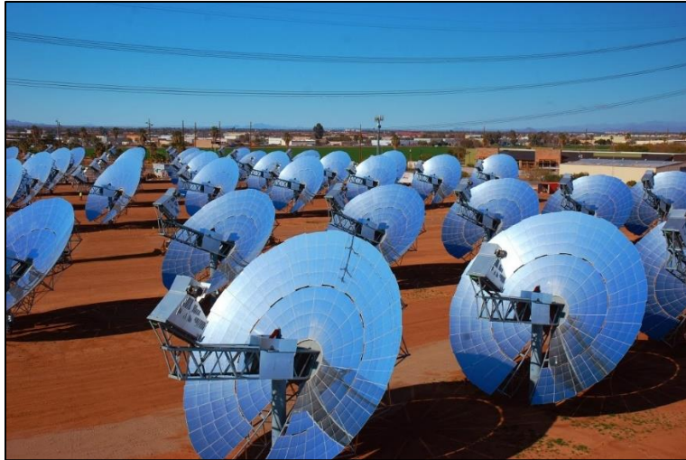
Figure 7: Parabolic dish power plants 7
