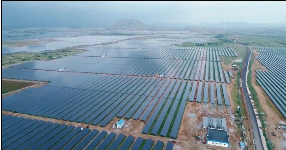
Figure 15: Pavagada Solar Park 16
